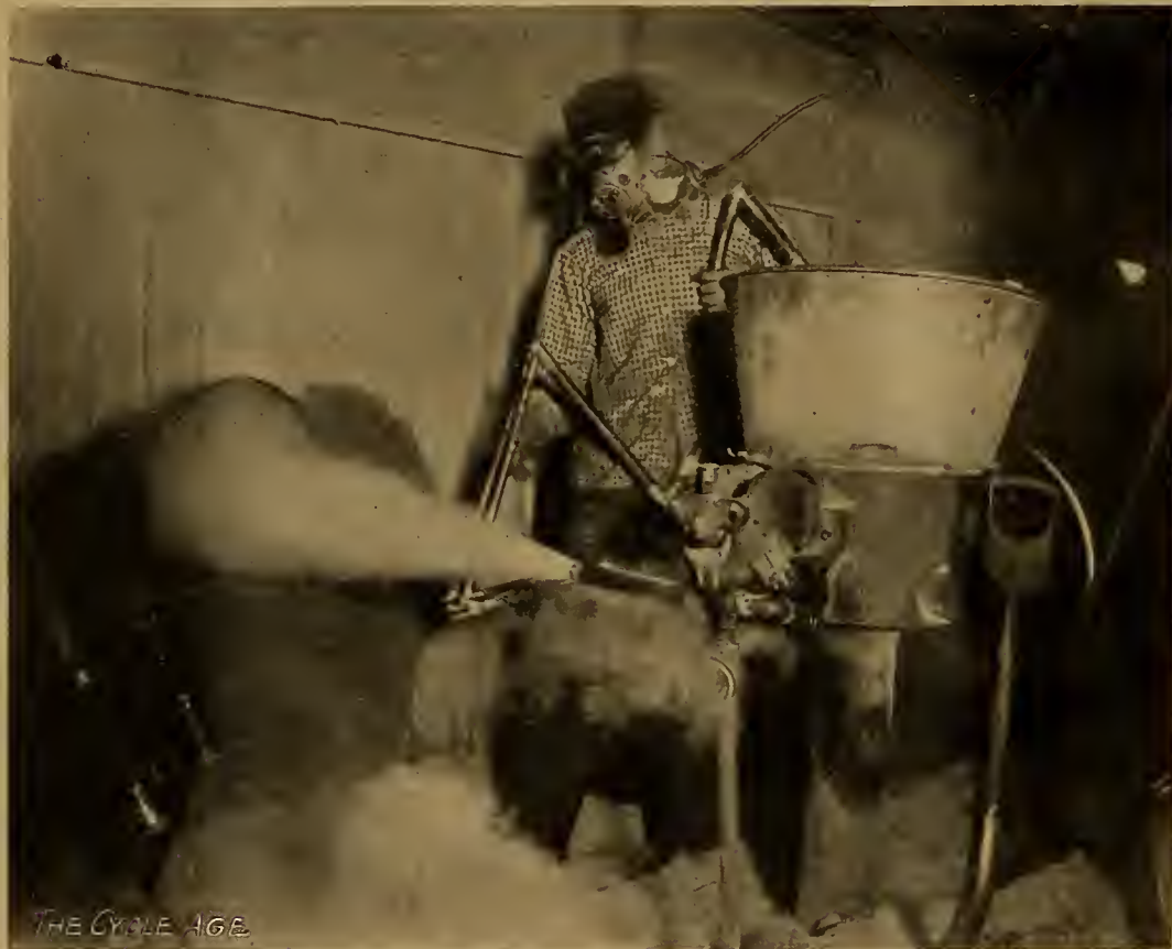
WET SAND BLAST IN OPERATION IN FANNING FACTORY
